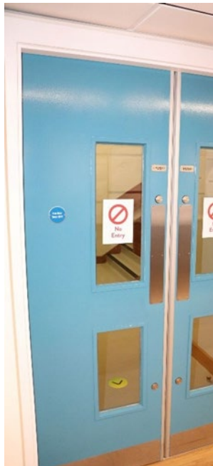
No entry stairway
