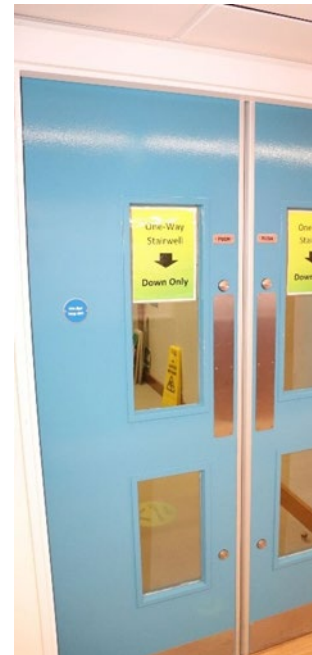
Down stairway entry
